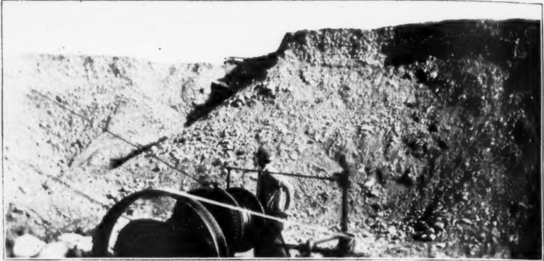
The Hoist Operating The Drag Scraper.
